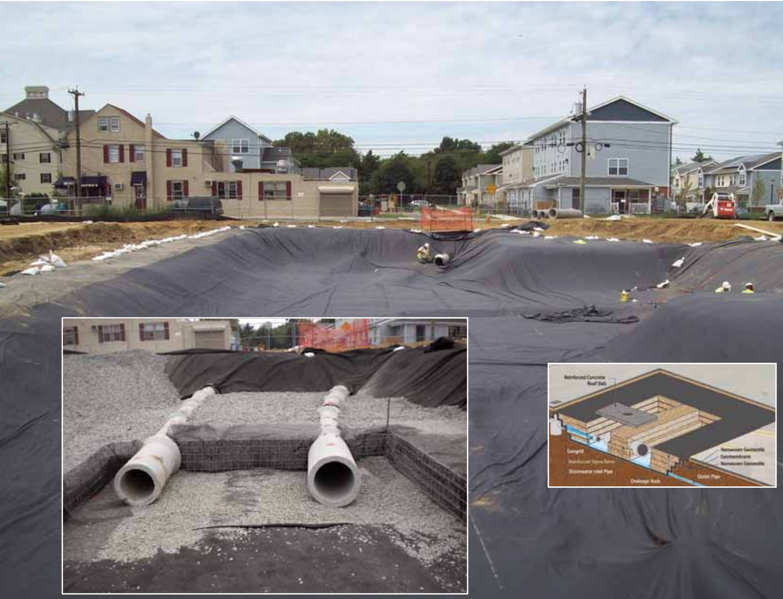
PVC geomembrane installation over underground chamber. Inset: Perimeter wall construction at pipe penetration. Schematic of patented geosynthetic based underground stormwater detention system.
