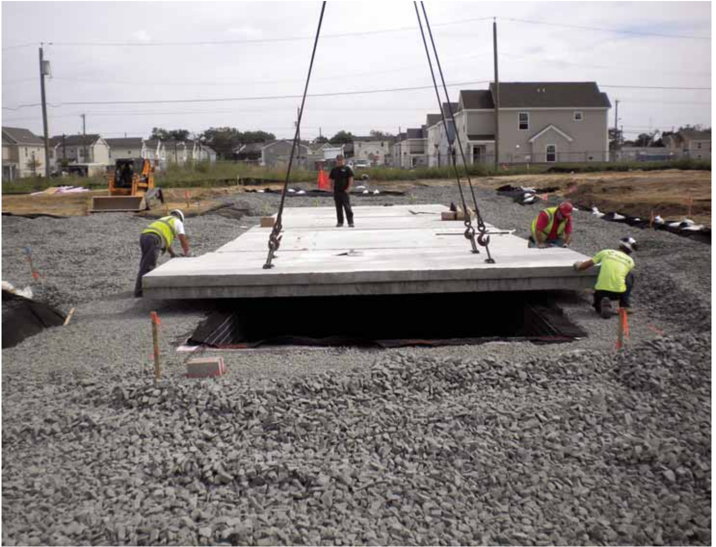
Stormwater detention system roof installation over chamber.
